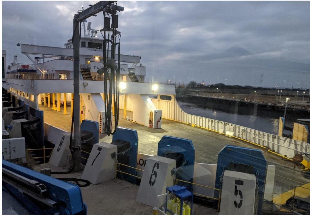
Figure 5. M/V CAPE HENLOPEN at Terminal
